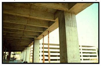
choice, pan joists with wide beams. This system is similar to the filigree system in that the weight of the slab is reduced by introducing voids into them with the pans in order to create ribs. The filigree system might have ended up cheaper since no additional form work is need during construction but structurally the designs should be comparable.
